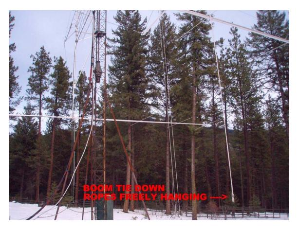
\_\_\_\_ Repeat on all four tie downs and confirm that all tie downs are properly hanging freely from the boom before exiting the antenna clearing.
