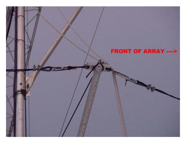
\_\_\_ The freely hanging tie-down lines are now flipped so they are both hooked around the FRONT of the fiberglass spreaders on the lower yagis.
