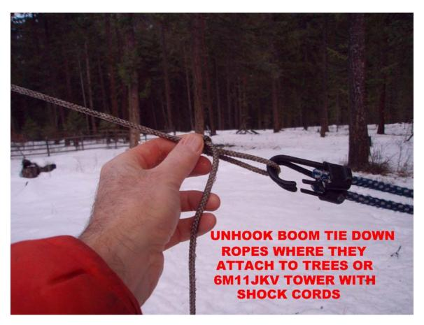
\_\_\_\_ Start out by releasing the tie-down lines where they are secured to the anchor objects (trees or tower). Drop the rope to the ground so it remains near the tie-down point.
