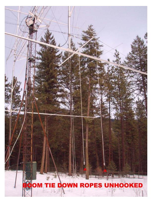
When unhooked, the tie-down ropes hang freely down, one on the FRONT side of the array and one toward the BACK of the array, with the white fiberglass spreader in the center of the lower yagis separating them.
