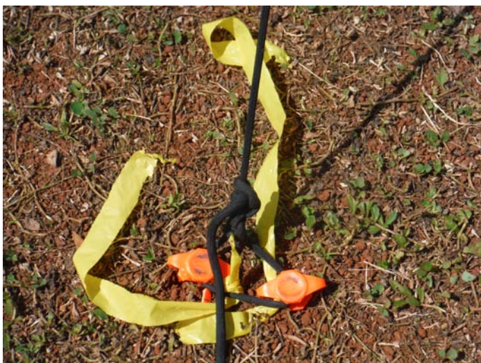
Using two spikes for mast guy anchors in the loose soil
