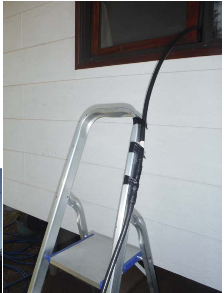
Feedline supported to just reach the amp through the window
