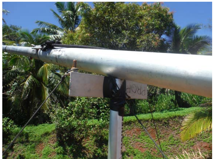
Prop turned upside down to use the base to support the mast.
