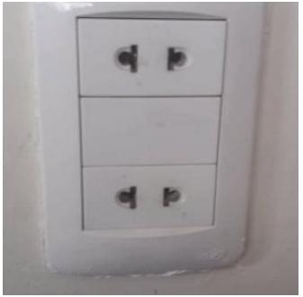
The AC outlets in the rooms were not wired with a ground. The outlets only provided two conductors - the 230 VAC and a neutral wire. So, it was necessary to add a separate ground for my equipment.
